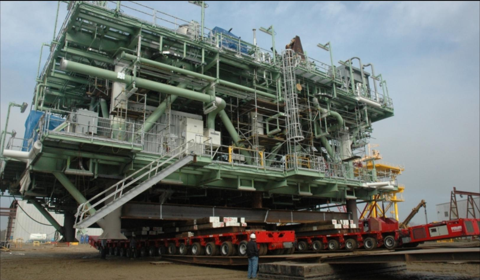
This job was a challenge due to the shallow water slip the barge was docked in. The barge height was 5' above the bulkhead so Berard engineers went to work designing and building a ramp system to move the 900 ton compressor onto the barge. Using 34 axle lines of Goldholfer transporters, the move was successfully completed on time and in a safe manner in only one day.
